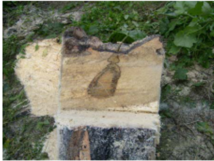
Figure 2: Section of palm to show drill hole plugged with forest cut plug (removed) to show decay.
