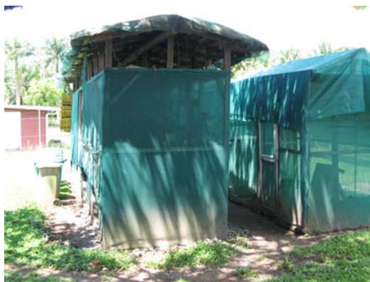
Figure 20. Part of Dami entomology section insectary with raised roof and sago frond thatching.
