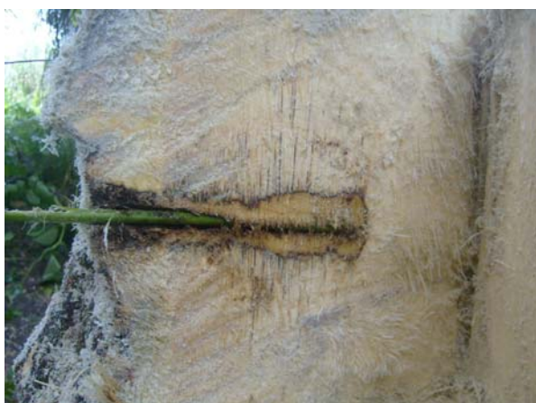
Figure 3: Drill hole plugged with palm nut (nut removed to show minimal decay). Note - the drill angle is incorrect in this photo as the section of palm has been removed for photography.
